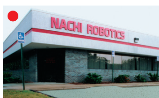
NACHI ROBOTIC SYSTEMS INC. (U.S.A.)
